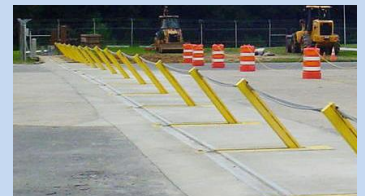
Electric Cable Trap. Source: RSSI
